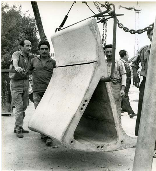
Images: (top) Sergio Prego, after Miguel Fisac's original drawing for Center for Hydrographic Studies, digital manipulation, 2019. Courtesy the artist; (bottom) Bone beam ready for installation during construction of the Center for Hydrographic Studies, Madrid, designed by Miguel Fisac, 1961. Courtesy Fundación Miguel Fisac
