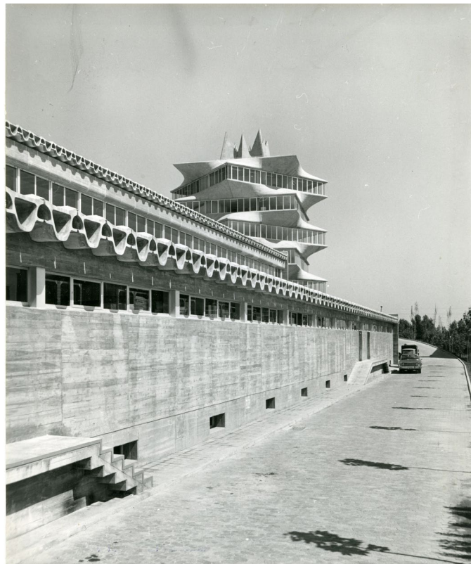
Images: (top) Jorba Laboratories under construction, Madrid, designed by Miguel Fisac, 1965. Courtesy Fundación Miguel Fisac. Photo: Portillo; (bottom) Exterior of Jorba Laboratories, Madrid, designed by Miguel Fisac, 1965. Courtesy Fundación Miguel Fisac
